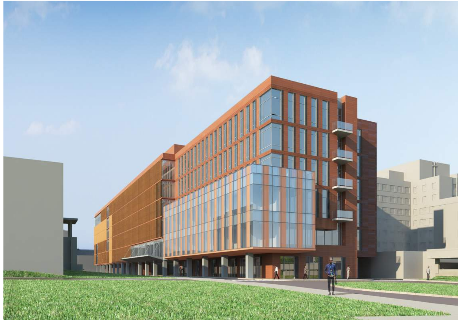
VIEW LOOKING AT NORTH EAST CORNER
