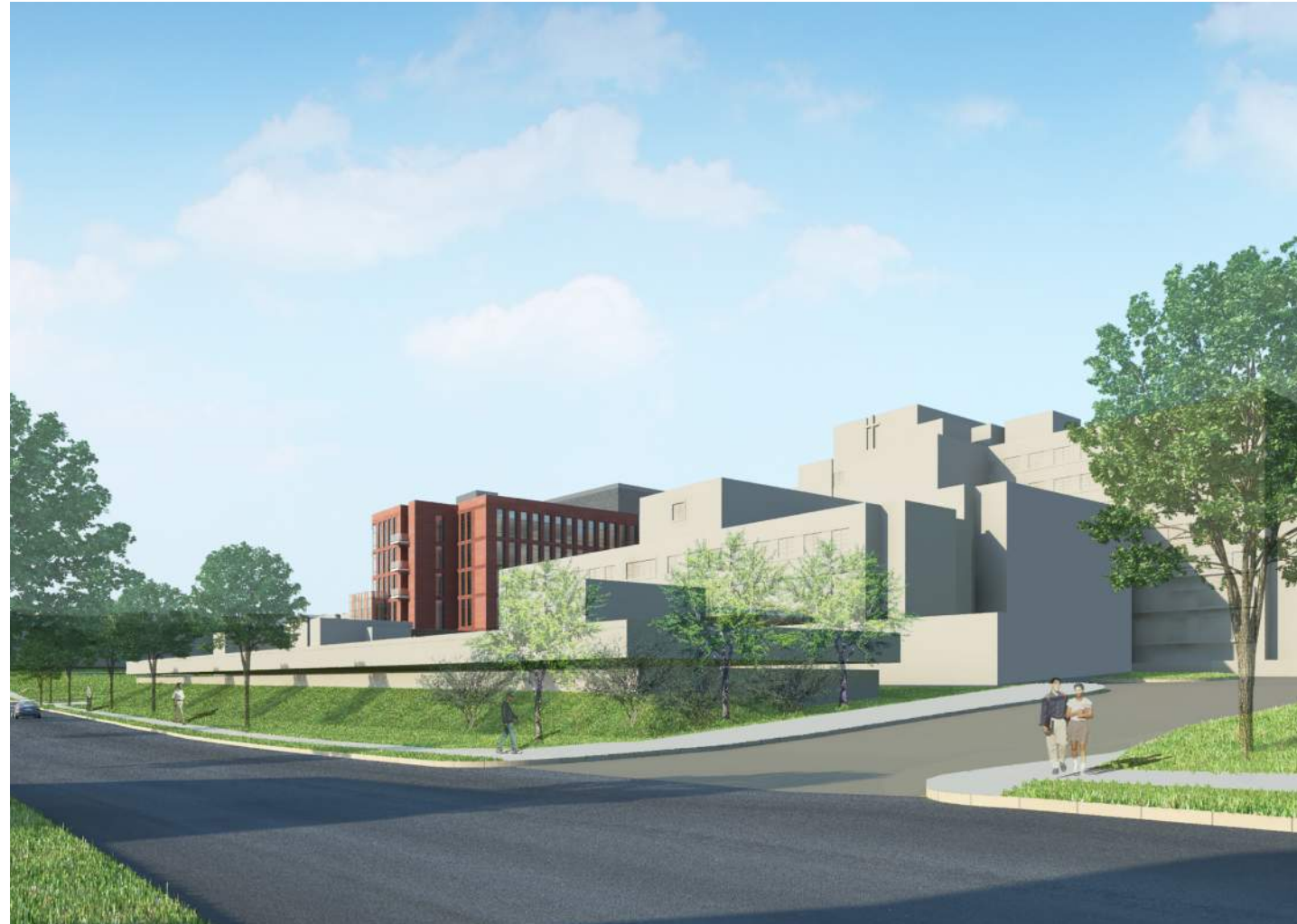
VIEW LOOKING AT NORTH WEST CORNER
