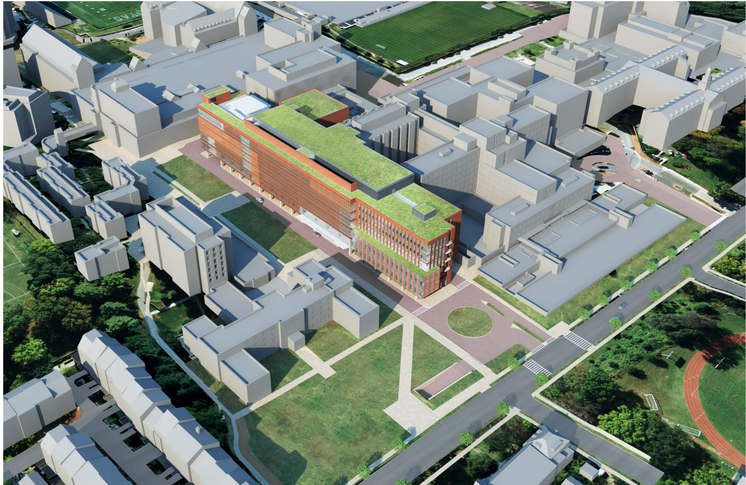
AERIAL VIEW FROM NORTH EAST
